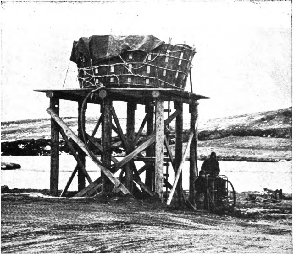
Figure 158. Water supply from stream.
